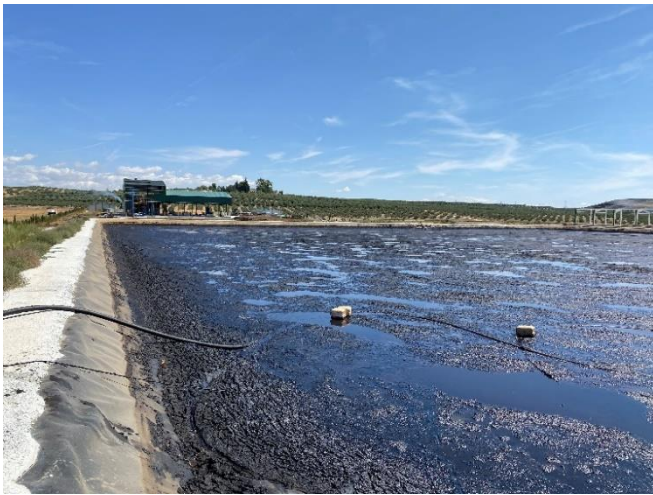
Figure 11: Aceites Guadalentín Facilities
