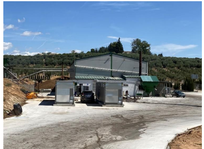
Figure 2: Aceites Guadalentín Facilities 2
