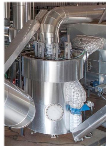
Streekpellets white pellet plant, The Netherlands, 2018 - 2020 Capacity: 10 kton/a
