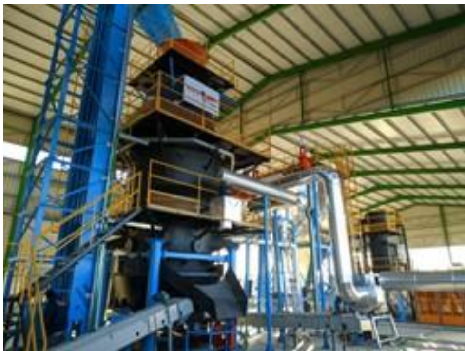
Figure 2: Aceites Guadalentín gasification plant to transform olive pomace into energy and biochar
